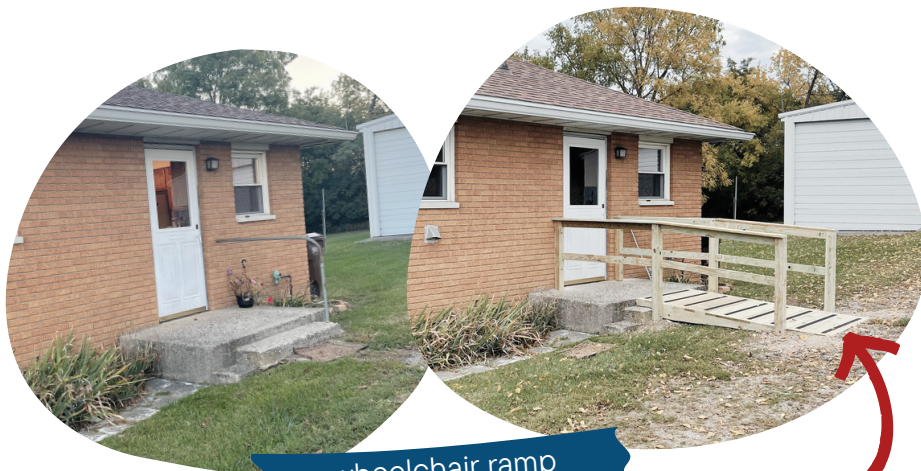
wheelchair ramp installation
